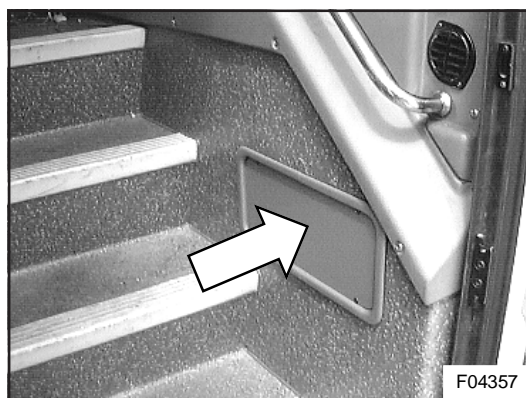
Figure 2: Access panel in the stepwell of the entrance door
