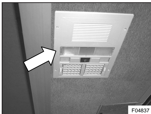
Figure 27: Control panel above passenger's seats
